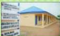
Completed Project at Okitina Primary School Gbagbe, Lagos
